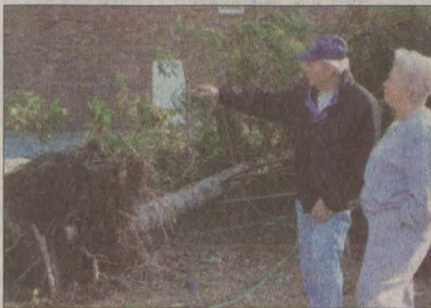
This carport collapsed in the wake of 70 mile an hour winds during Wednesday's storm.
