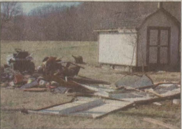
The storm destroyed one storage building in Nell Conley's back yard, while leaving another standing only feet away.
