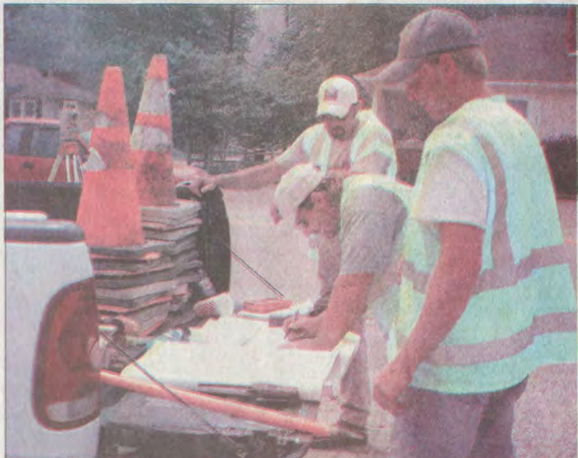
photos by Mary Music Surveyor Mike Rowe, center, reviews plans concerning the North and South Lake Drive "makeover" project with surveyors Forrest Newsome, left, and Danny Cooley. The men work for Mountain Enterprises, which was awarded the $575,663.94 contract.
