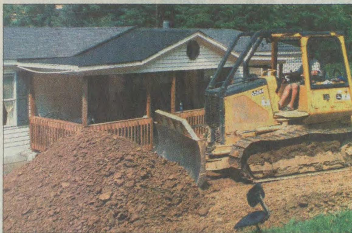
FEMA funds at work at the Stevens residence on Abbott Creek.
