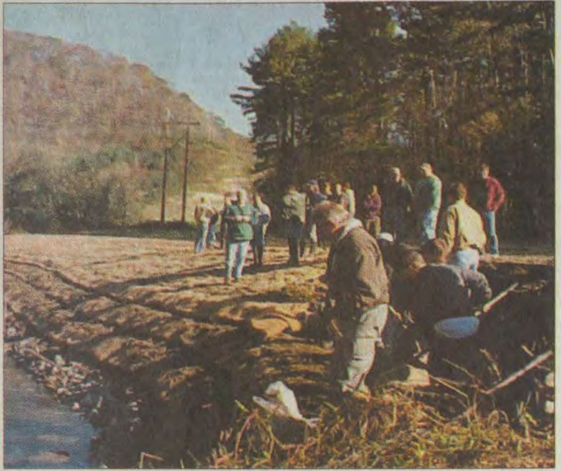
Participants in the soil bioengineering workshop are shown installing soil blankets and layers of willow cuttings between the soil blankets.
