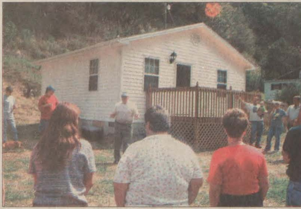
The Floyd County Fiscal Court and the Floyd County Area Technology Center held an open house to recognize all of those involved in the construction of a home for Haskell Hall in McDowell.
