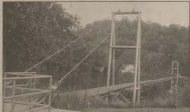
The new pedestrian bridge that spans Levisa Fork, at River, is the longest fiber-reinforced composites, plastic, suspension bridge in the world.
