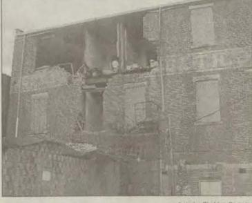
photo by Sheldon Compton A large portion of the back side of the old Hobb's building in downtown Prestonsburg was torn away by strong winds during Wednesday night's thunderstorm. The building may now have to be torn down as a result of the damage which left much of the inside exposed and many sections hanging and threatening to
