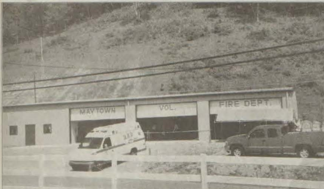
The new Maytown Fire Department facility located at Langley
