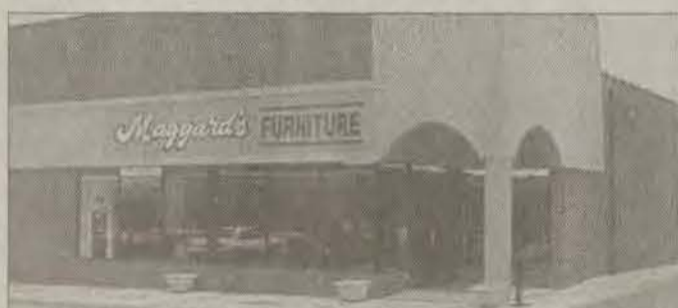
The new Maggard's Furniture Store is located on East Court Street, in Downtown Prestonsburg (formerly the Sears Store).
