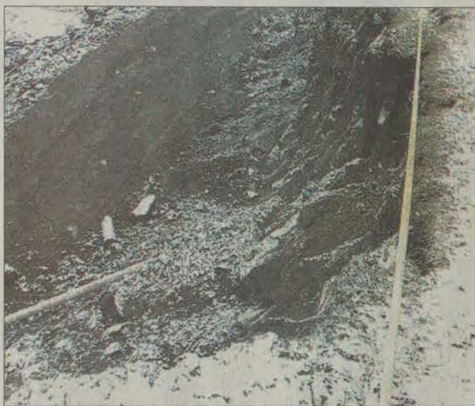
A rain-induced slide in a construction zone at the northern entrance to Jenny Wiley State Resort Park left about 35 households without water.
