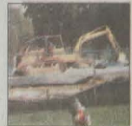
Preparing the site for a new building on the PCC campus
