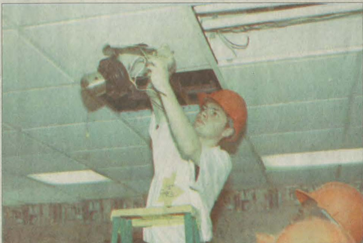
Students from the Carl D. Perkins Job Corps are taking part in Volunteer Week by volunteering their time and skills to various agencies throughout Floyd and Johnson counties. Here, Elijah Davis repairs a light fixture in the Property Valuation Administrator's Office in the old courthouse. Davis was one of 11 students from Tim Young's class that did work in various parts of the courthouse on Thursday. (photo by Willie Elliott)
