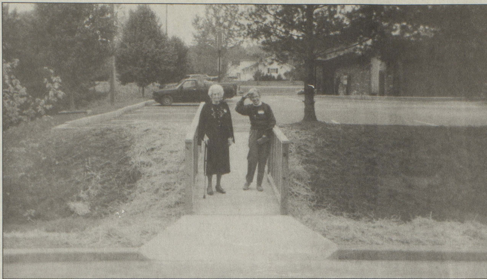
Orbie Vaughan and Eloise Collins were the first residents of Highland Terrace to stroll across the new bridge between the apartment complex and Wendy's Restaurant in Prestonsburg. The city recently had the bridge constructed.
