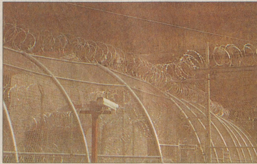
Should Otter Creek Correctional Center convert to medium security in its proposal to bring in 600 out-of-state inmates, a second razor-wire fence like the one above would be constructed around the prison to beef up security. Otter Creek, which was plagued by walkaways in its early years, has had no escapes since a security upgrade was completed in 1997. (photo by Ralph B. Davis)
