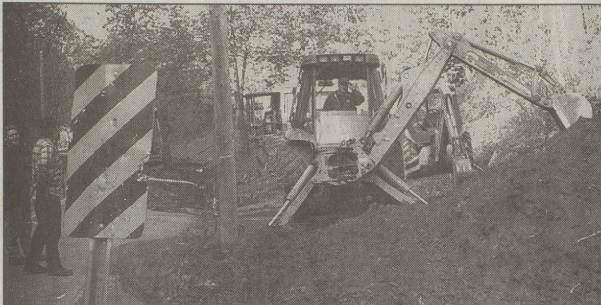
This driver is all smiles as he digs a ditch to install water pipes, but he is not pleased nearly as much as the residents of Bill Hall Branch who will soon be able to tap on to city water. (photo by Willie Elliott)
