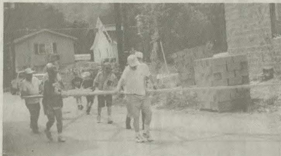
Church members carried roof trusses up the street to the building site.
