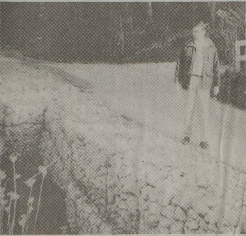
Road work at Slick Rock
