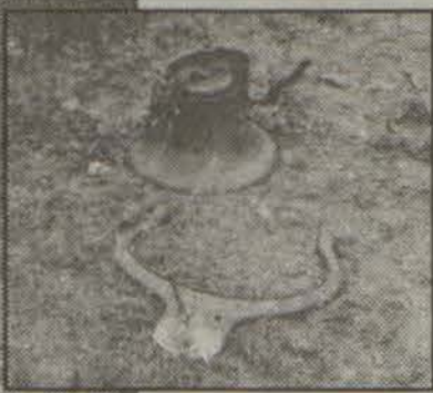
Damage was extensive to Parkway Baptist Church after an early Saturday morning blaze. Only the church bell survived the fire that was probably caused by an arsonist.
