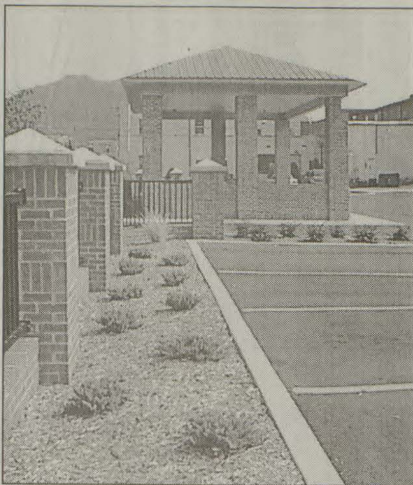
The new Town Center Parking Lot in Prestonsburg is located across from the Town Center Building on North Lake Drive. The stage area of the parking lot is used for free concerts. The parking lot is also the scene for festival fun in October when the Jenny Wiley Pioneer Festival brings activities to the lot. (photo by Janice Shepherd)
