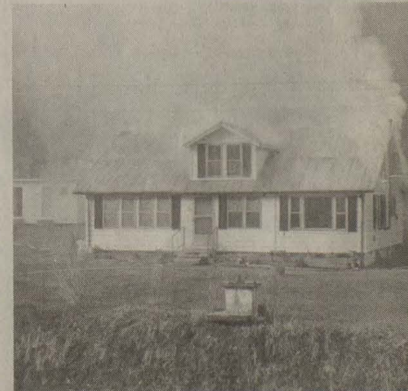
Crider home damaged by fire
