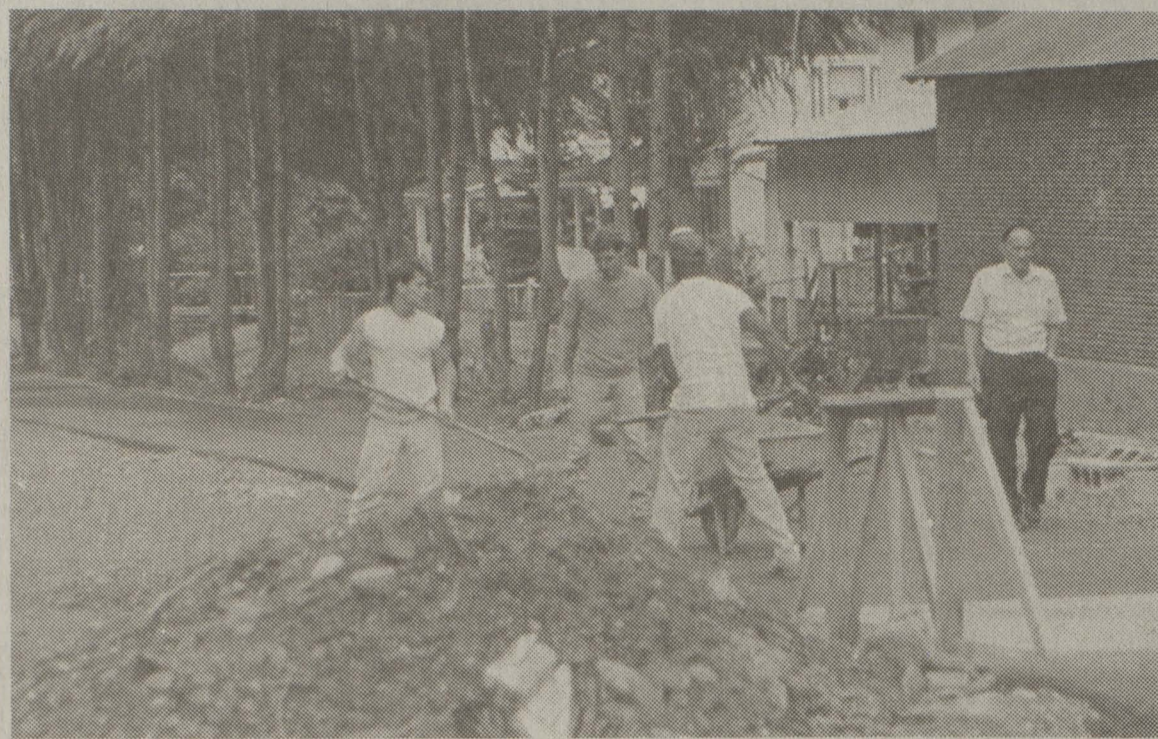
Work continues on walking track
