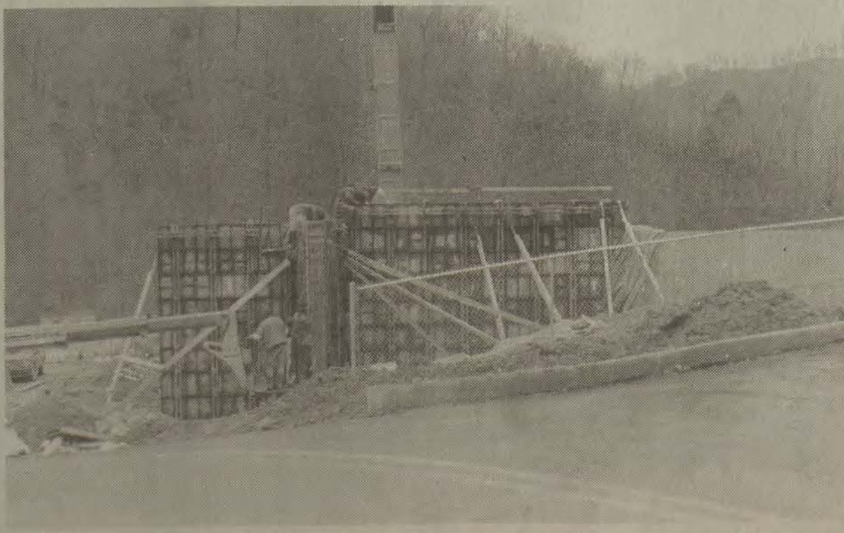
Work progressing on gym
