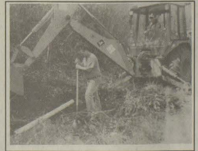
250 MILES OF WATER PIPE
