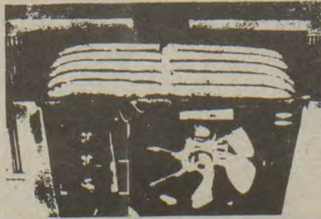
Some units have spine fins. Despite their coniferous appearance, do not attempt to straighten them.
