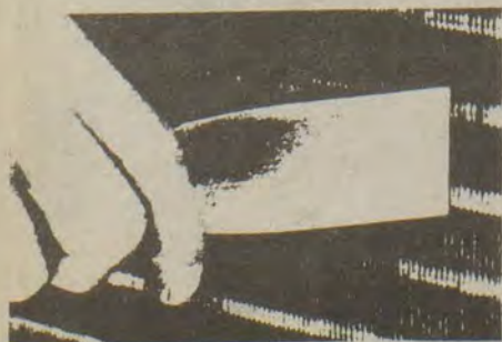
Use a putty knife to restore the space between fins. No two fins should touch one another.
