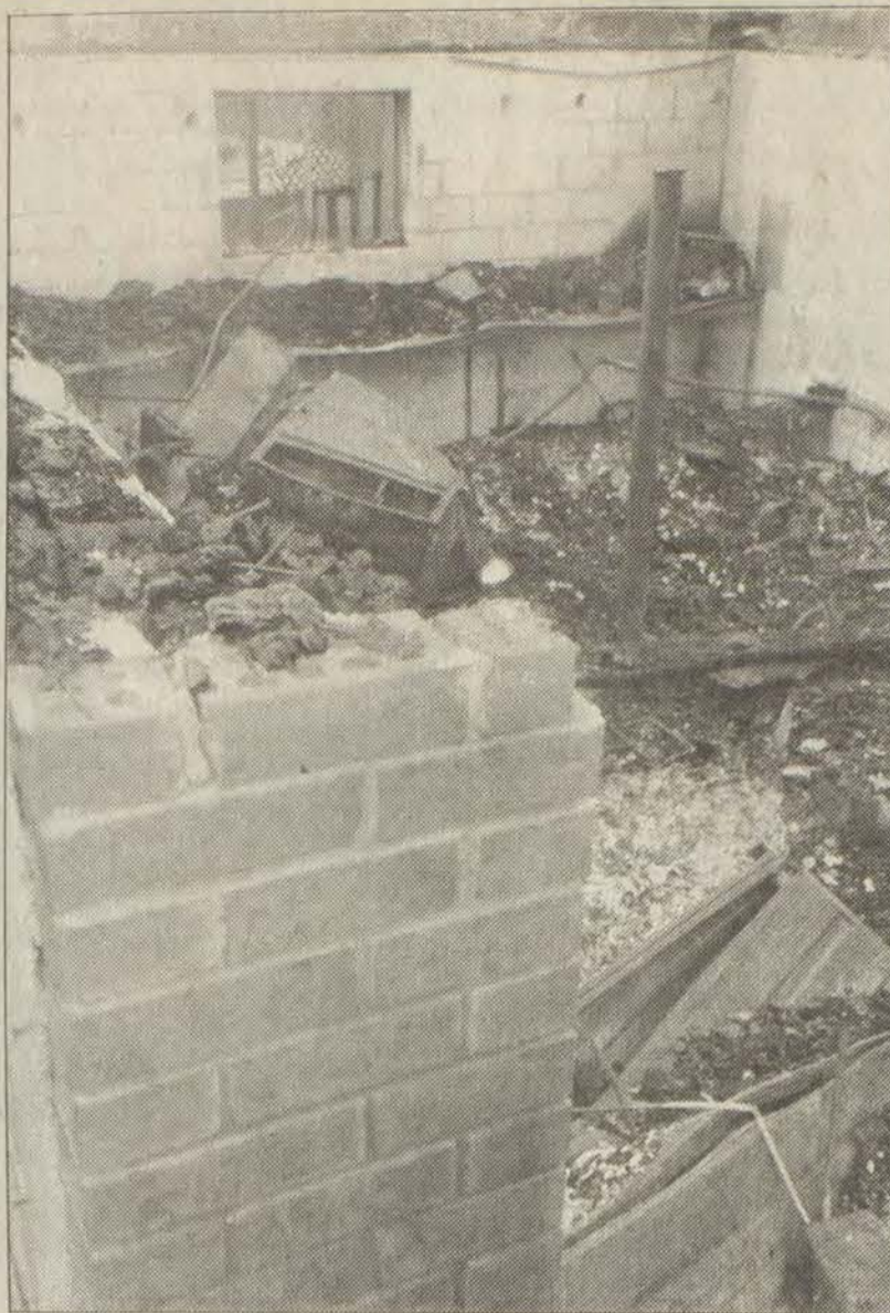
Home Destroyed By Fire
