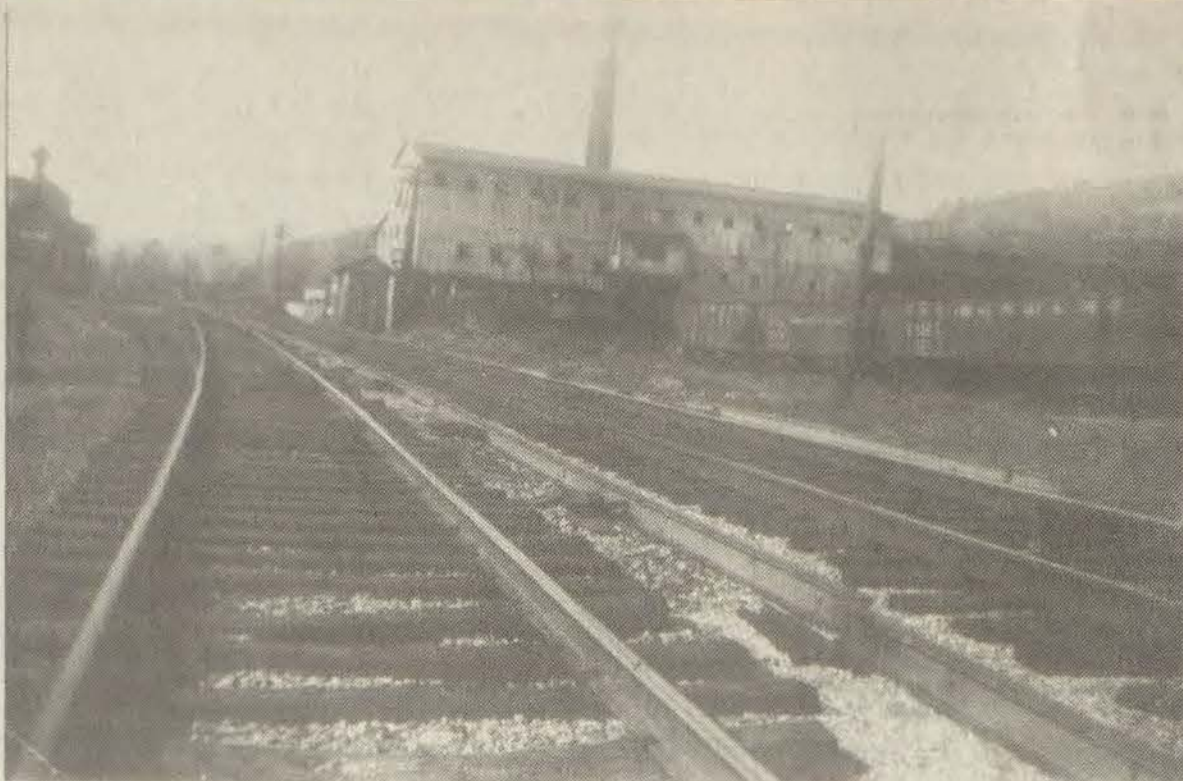
A rare tornado touched down in Auxier in the 1920s, doing considerable damage to the coal tipple, shown here with one end cracked.
