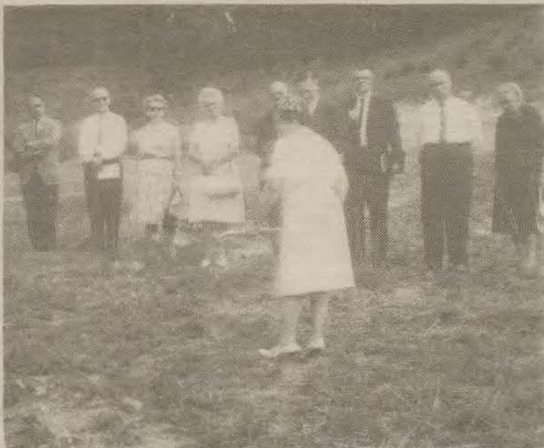
A groundbreaking ceremony in May 1965 for the First Presbyterian Church in Prestonsburg is shown above. Ruth D. Sowards, with shovel, actually broke the ground; she did so because she had the longest membership in the church at the time. Also pictured are Dr. George P. Archer, mayor; Lon B. Rogers of Pikeville, Mrs. Frank H. Layne, Mrs. E.R. Burke; William Bunting, an elder; James E. Goble, an elder; Edford Clark, an elder; Rainley White, an elder; Mrs. Mae Ford Hyden and Sowards.
