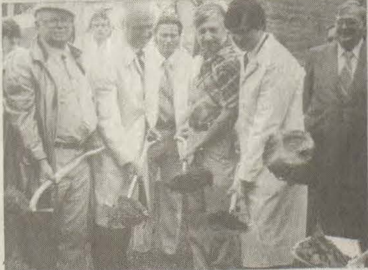
1979 Groundbreaking for Ulysses to Inez Highway and Ky. Rt. 3 resource recovery roads.
