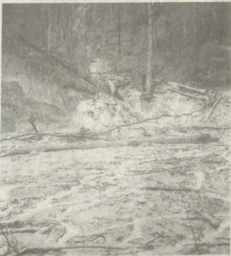
Rains Cause Mudslide
