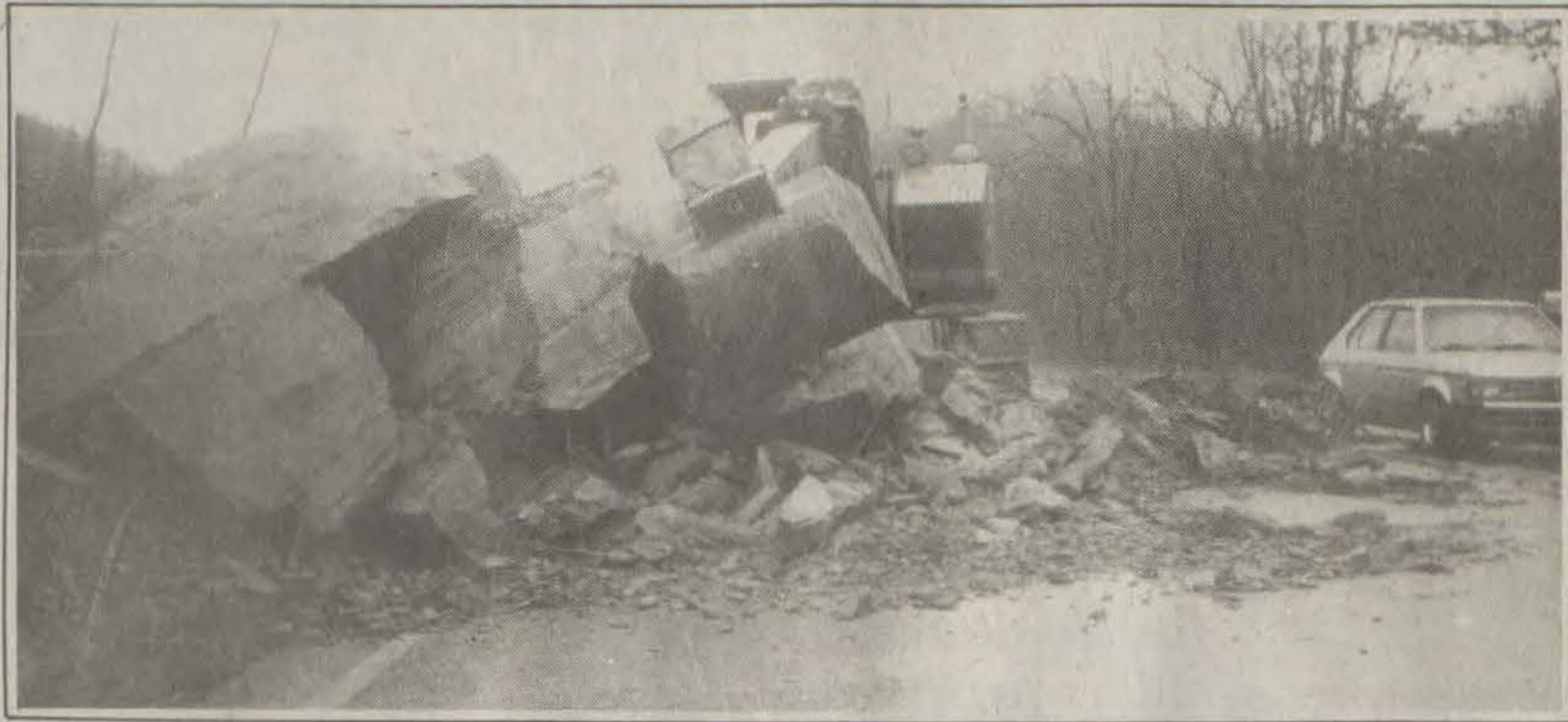
Rock Slide Blocks Road
