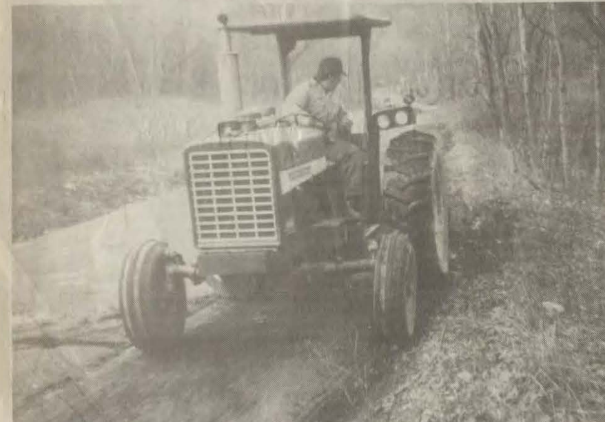
Do-It-Yourself Road Repair
