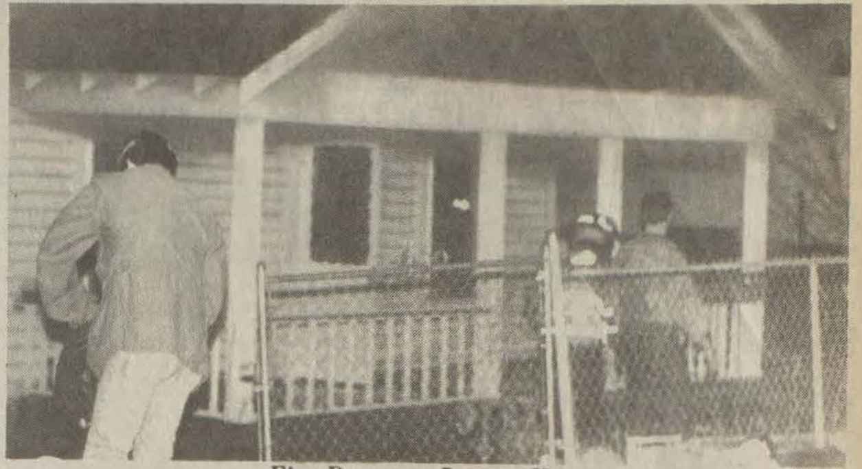
Fire Damages Lancer Home
