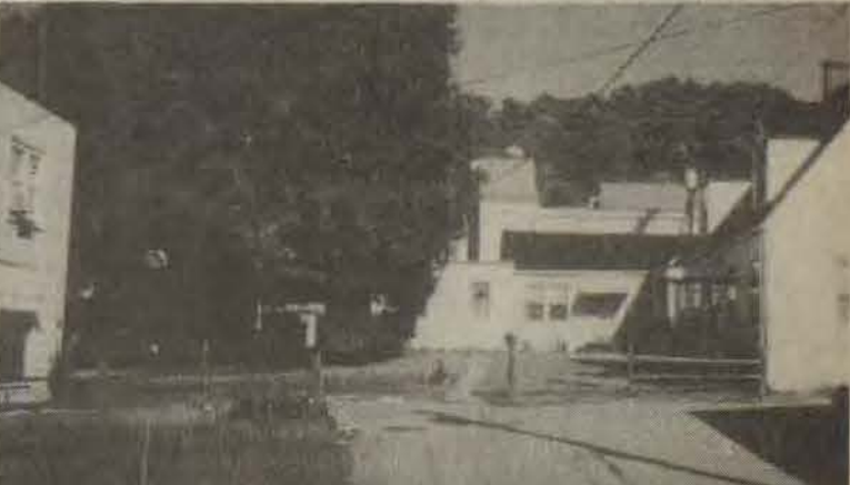
FRANCIS COURT, PRESTONSBURG—Excellent location for residential and/or commercial use of income. Property consists of 135' x 116' ± lot, two houses, and 2-story concrete block building with apartment up and business down. A total of 5,000 ± sq. ft. of usable space. Call for complete details.
