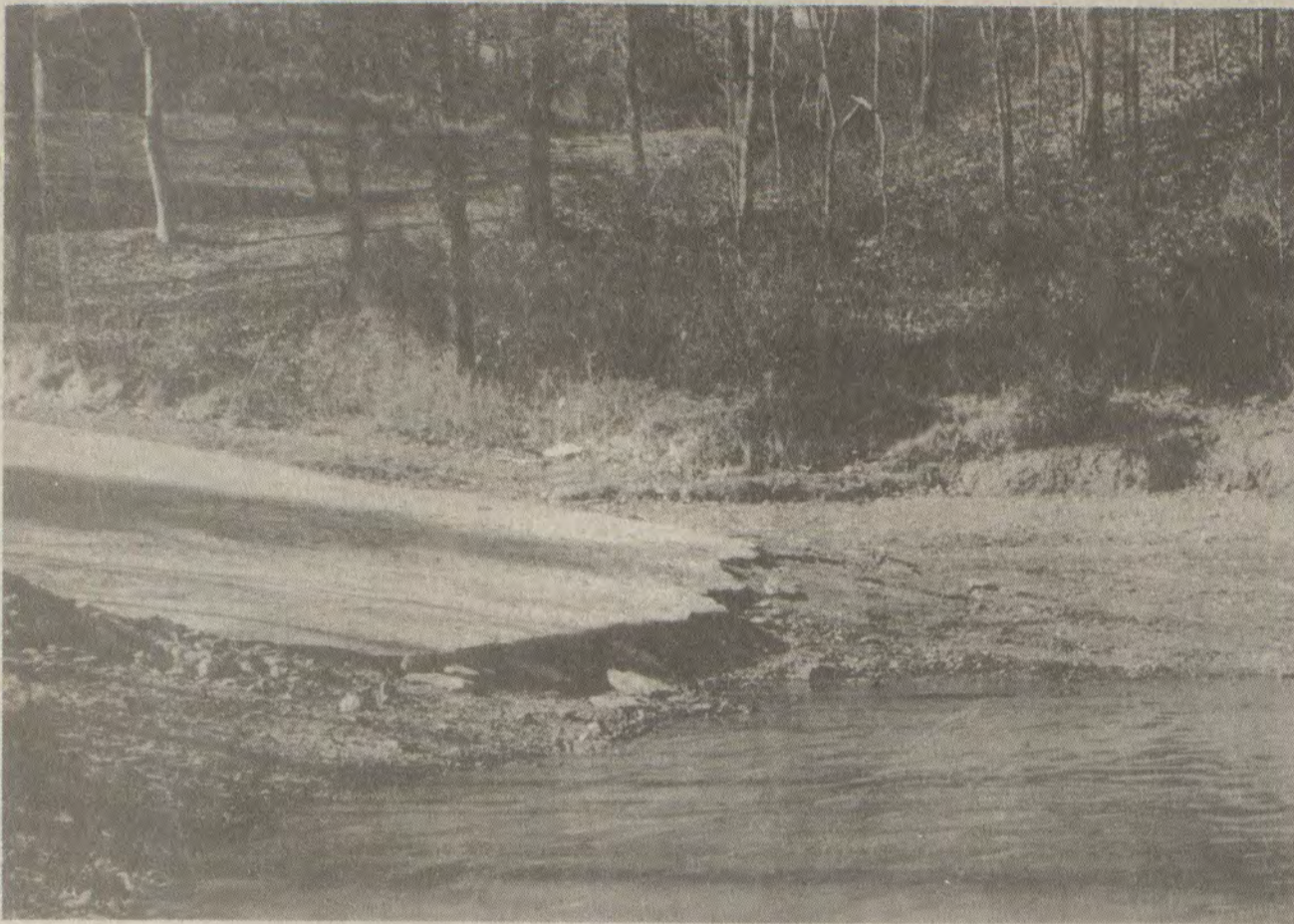
GOBLE BRANCH BOAT RAMP, at Dewey Lake, ends with an unwelcome surprise for unwary drivers—a foot-high drop to the water. Tire tracks on the far bank show where some drivers have bypassed the ramp. The drop-off will disappear when the lake fills up to its summer level.
