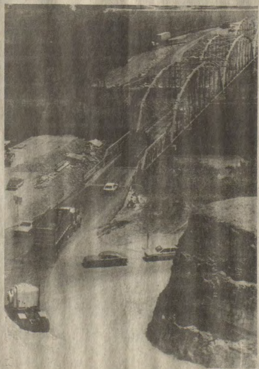
THIS SMALL MOUNTAIN OF ROCK at the intersection of KY 1427-1428 has some Abbott Creek residents fearing an increase in traffic accidents there. Though some want the obstruction removed, state highway department officials insist that the problem will end when the new Cliff Bridge opens and changes the angle where the roads intersect.
