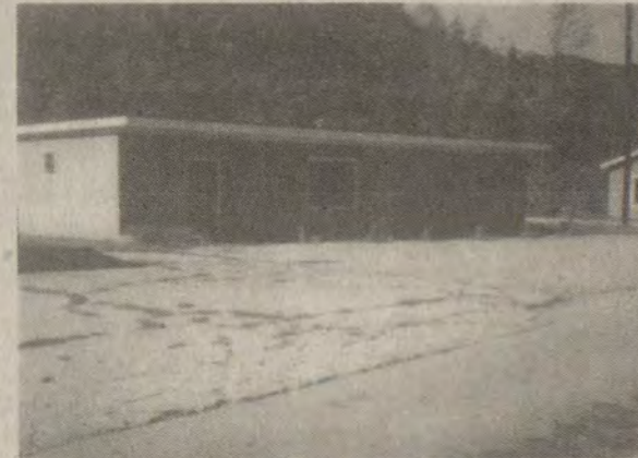
80x75-ft. lot with 28x50-ft. block building, set up for laundrymat in Goble-Roberts Addition. Can be changed to another type business.
