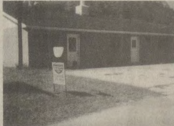
72x100-ft. lot with 30x50 frame building. Commercial property now being used for church. Come see, come buy.
