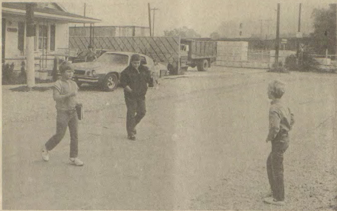
PARENTS' FEARS for their children's safety, and the right of a merchant to use his property the way he wishes, have come into heated conflict on this street corner in West Prestonsburg. The issue centers on a new, 50-foot section of sidewalk (in background of picture), where Main Street meets Railroad Avenue.
