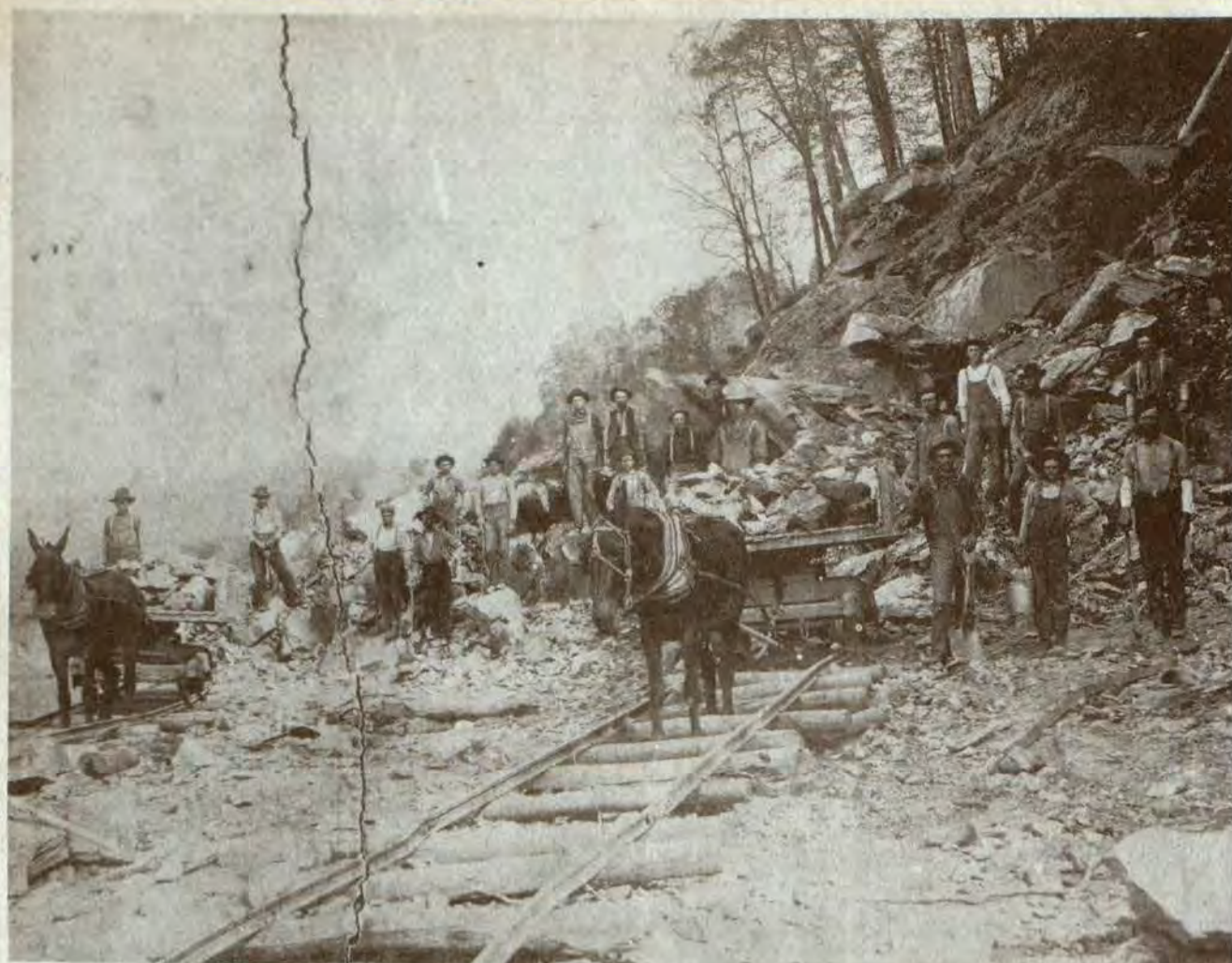
BUILDING THE RAILROAD AT EAST POINT IN 1903... While this same cut was being made holes were drilled to blast away the rock, one shot failed to detonate and a man named Burke was killed by the delayed explosion. Identified, from left—Mont Lilly, East Point, driver of dump cart; Lonnie George, East Point; two unnamed Magoffin county men; Ike Hurd, "Red Cap" Sparks, Tommie George, Ad Wilcox, Albert Barnett, foreman, two Magoffin county men, Jeff Moles, driver of second cart, three unidentified men, Henry Burke, Pitt Harmon, water-boy, Grant Burke, unidentified man, Fox Dale, Add Wilcox. (Photo and information by Warden Auxier, Inez Rd., Paintsville, Ky.)
