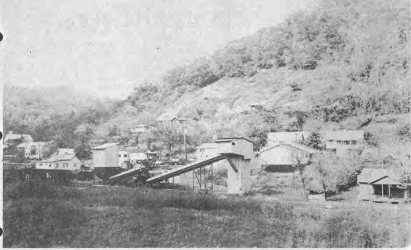
NESTLED AMONG HOUSES in the community of Dinwood, just south of Martin, a coal tipple operated by Dinco Coal Sales Inc. won the right to resume operations last week, an administrative law judge ruling that the U.S. federal Office of Surface Mining, which shut the plant down in July, does not have jurisdiction over the tipple. An OSM inspector had cited Dinco for operating the tipple within 300 feet of several residences without getting the waivers required by law. Several area residents have long complained of noise, dust and diesel fumes associated with the plant.
