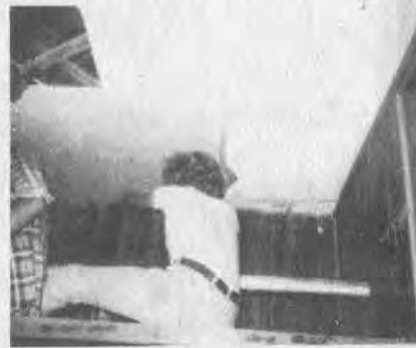
Interior Repair Work—Replacing damaged sheetrock and drywalling.
