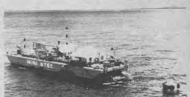
Mini-OTEC, the pilot plant off Kona, Hawaii, uses warm ocean water to produce electricity at low cost.
