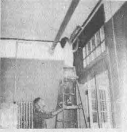
Participants were instructed in proper use of ladders and scaffolding.
