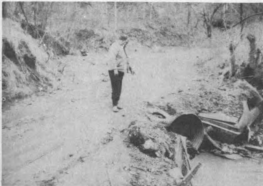
Deteriorating road in Boyd Branch of Prater Creek
