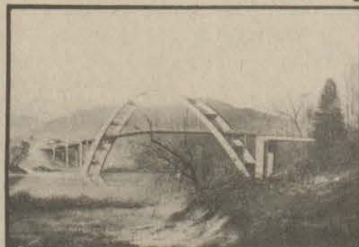
W. Prestonsburg Bridge
