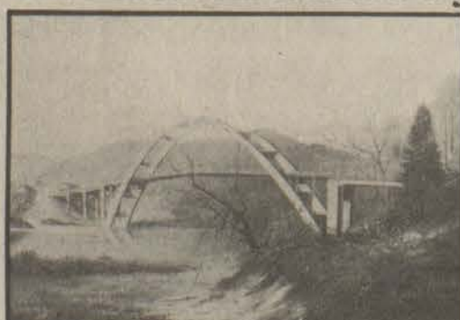
W. Prestonsburg Bridge
