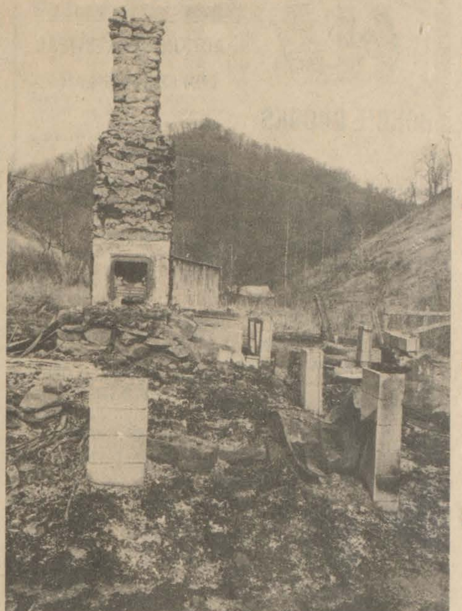
CHARRED FOUNDATION STONES and an old rock chimney are all that remain of the frame house which burned at Risner last Tuesday night as the result of apparent arson. The structure was owned by Mr. and Mrs. Whitts Click, of Risner.
