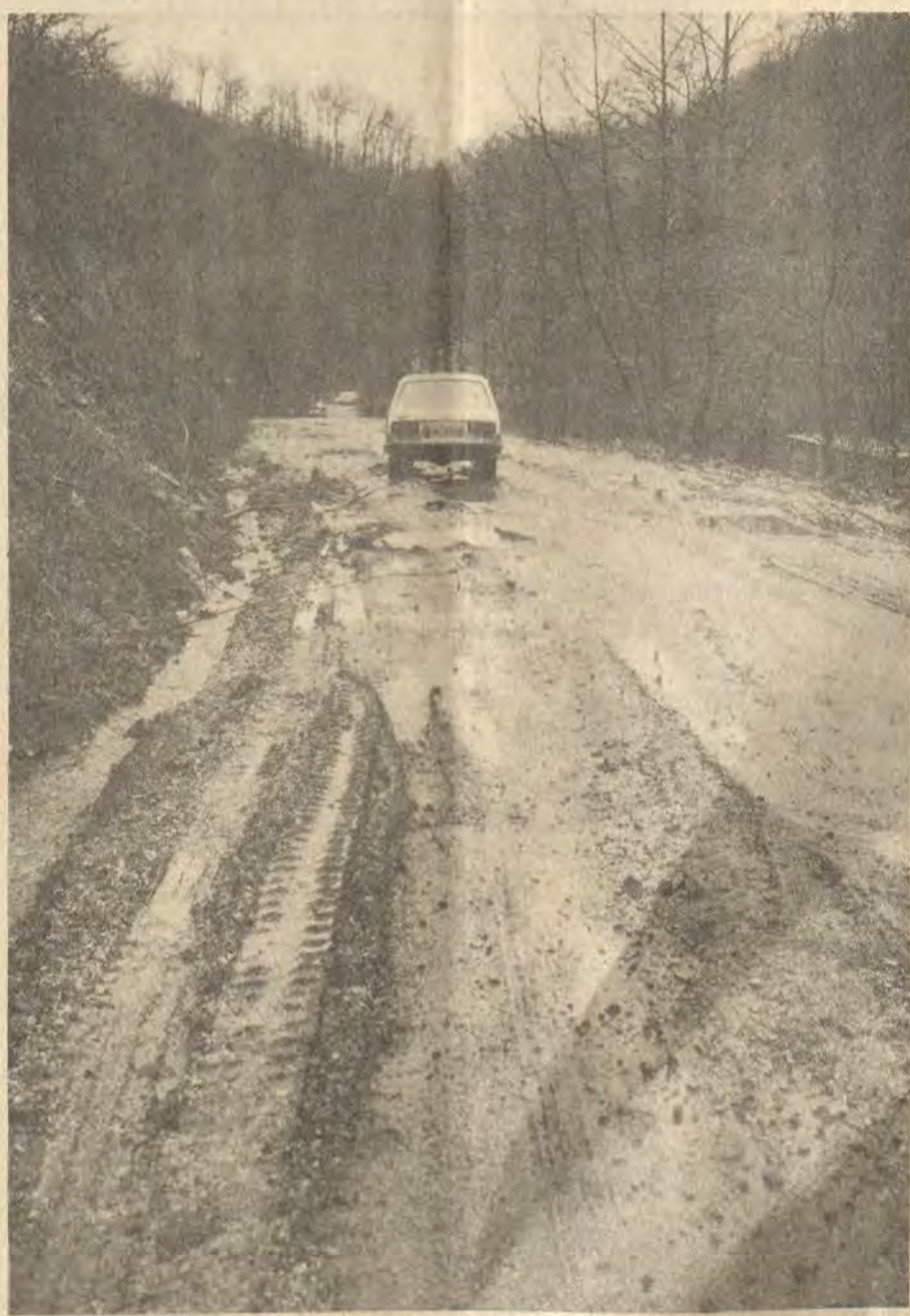
ROAD CONDITIONS in the Little Mud Creek section, typified by the accompanying photo, were the topic of a community meeting Friday night at the Spruce Pine school. Similar situations in various parts of the county are a source of concern for many Floyd residents. (See story, Section 2, Page 2.)
