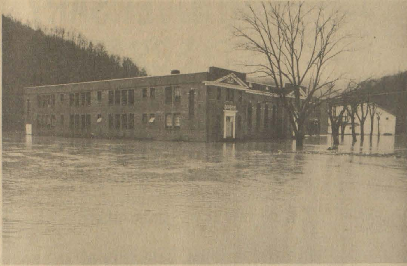
FLOOD WATER, the result of nearly three days of steady rain which swelled nearby Beaver Creek, surrounds the Garrett school and gymnasium in this photo taken Saturday morning.
