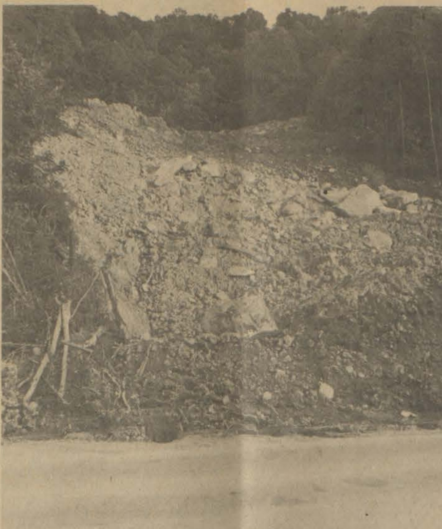
Many residents of the Martin-Maytown section are concerned by this large earth and rock slip which borders KY 80 on the section of that road below Maytown known as the "Warco straight." Sizeable boulders protrude dangerously from the steep slip which could become even more unstable with the arrival of wet weather.
