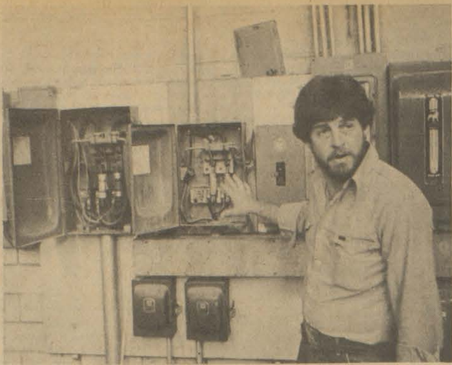
Jim Osborne, at a meeting of Parents for Better Schools, explains the danger of open electrical switch boxes, which were seen when the group toured the high school building here last Thursday. These boxes are located in the stage area of the gym.
