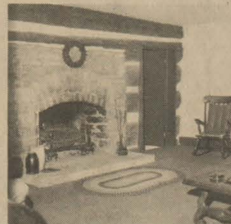
INTERIOR OF HOUSE
