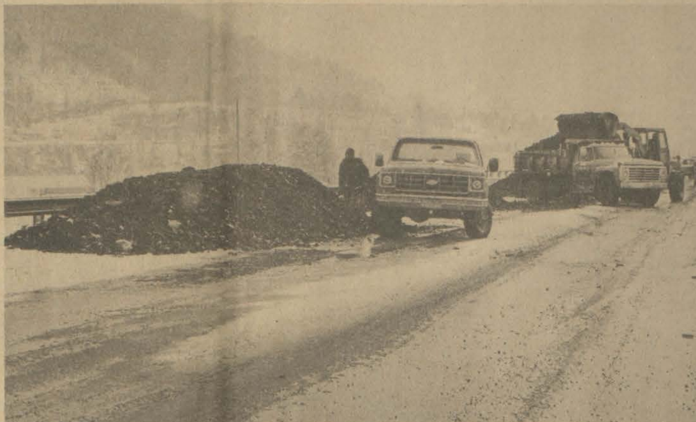
HIGHWAY CREWS work to clear lane of US 23 bridge at Allen where several coal trucks were forced to dump their loads Tuesday morning.
