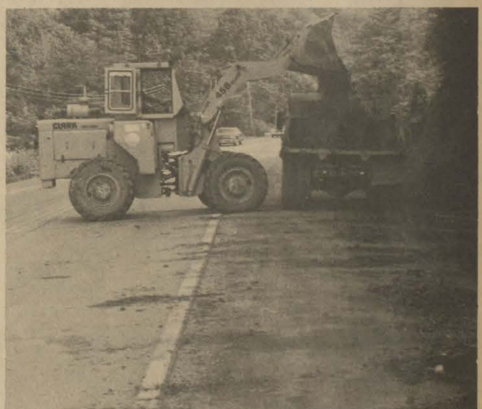
U. S. 23, between Auxier and Prestonsburg, has been the focus in recent weeks of highway crews engaged in ditching, installing drains and cutting weeds along the right-of-way.
