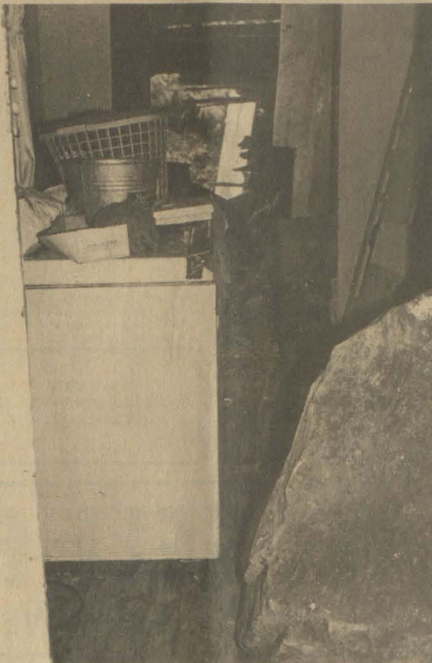
View of Mulkey residence shows where boulder came to rest after ripping a large hole in the back wall of the house, visible in background. (See additional photo elsewhere in paper.)
