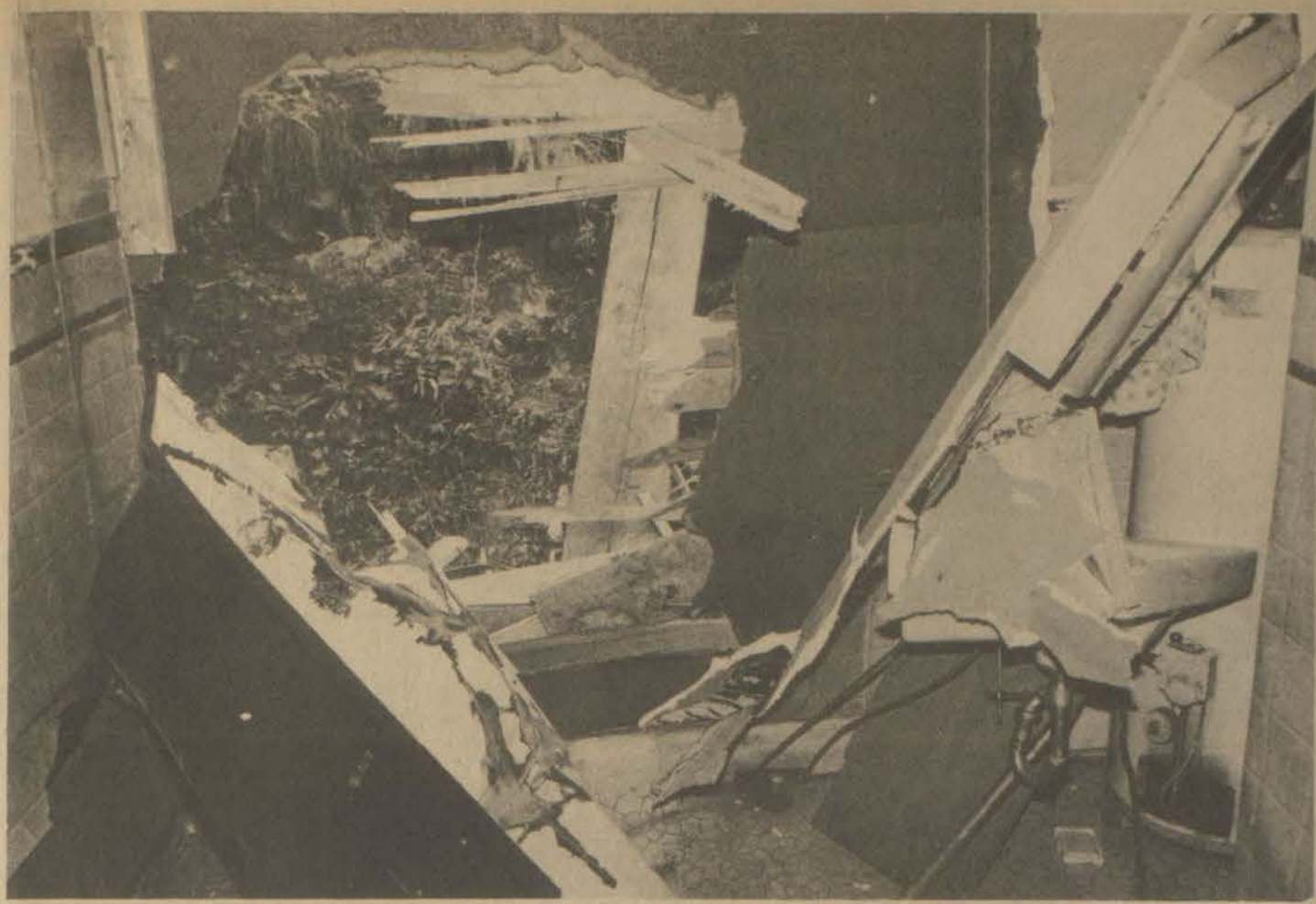
HOLE IN WALL and interior damage caused by a large boulder which rolled off the hillside behind the home of Bertha Mulkey, Thursday, is evident in this photo. (See story, Page 1)
