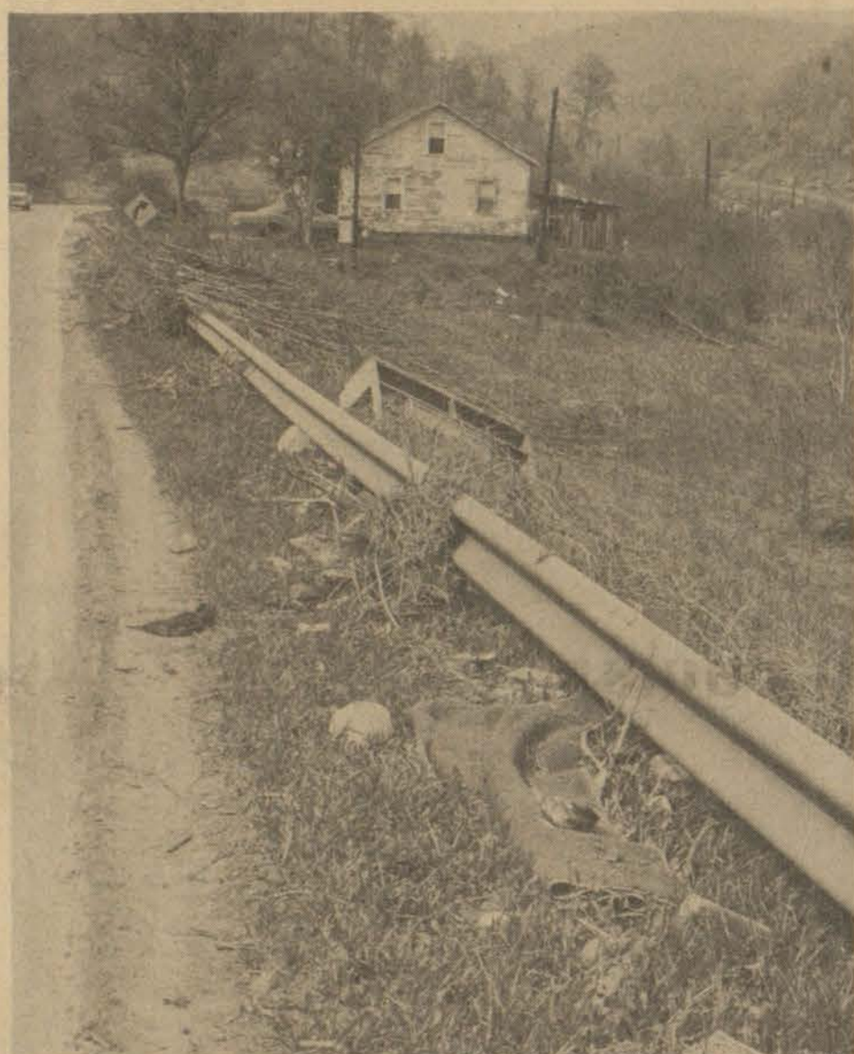
TRASH AND DEBRIS line the right-of-way of numerous roads and highways in the county, reminders of the recent flooding. Above photo was taken along the road which approaches Jenny Wiley State Park from US 23 south.
